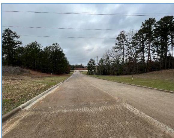
Facing Northwest along Willow Creek Dr.
