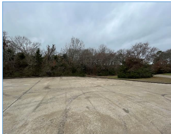
View from court facing SW towards R084341
